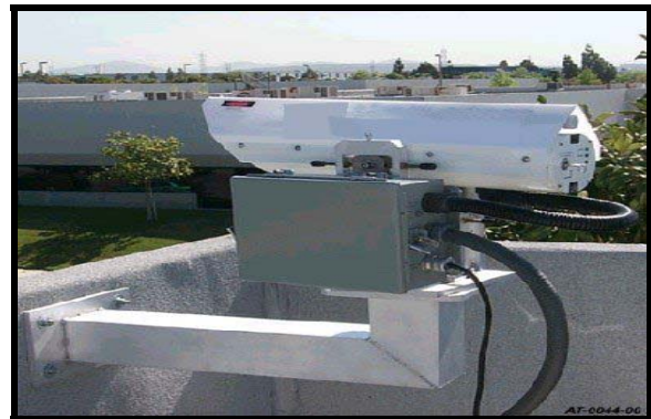
Figure 13: Extended Wall Mounting (using JMP and M062C)
