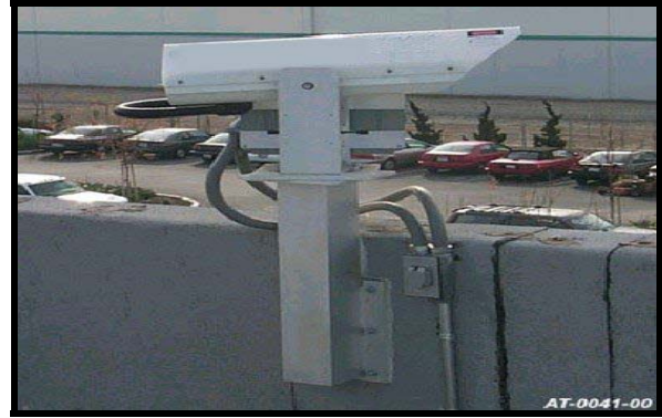
Figure 12: Wall Pedestal Mounting (using JMP and M054C)
